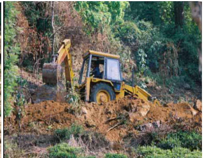
Leveling the Site
